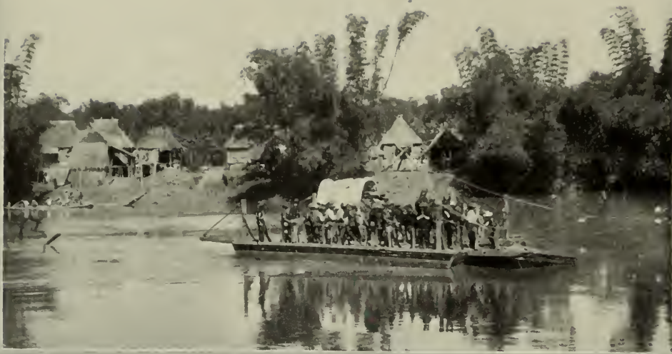
Flying Ferry near Arayat, Installed by Engineer Troops.
